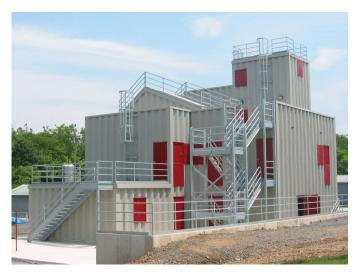
We held the responsibility for programming, design and construction administration for the Bucks County Burn Building. The training building is two stories tall, with a four story stair tower, residential section with an attic and singlestory annex. It features eight Class A burn rooms allowing firefighters to train with live fire. A va-
